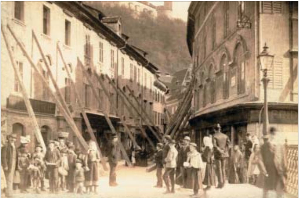
Figure 2: Demolished building at the end of Sv. Peter Street, today's Trubarjeva Street (Hefler, W., 1895, NUK). Buildings were not destroyed completely during the Ljubljana earthquake, but great damage was caused by falling chimneys, and walls and vaulted ceiling constructions cracked, particularly in those parts of the city where the structure of the ground was most vulnerable. Of 1,373 damaged buildings, only forty-nine were later pulled down. After the earthquake, a law was passed that required a suitable distribution of walls and the installation of iron reinforcing in the brick walls of new buildings.
