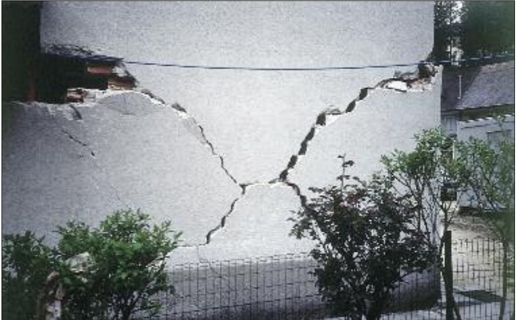
Figure 8: Typical damage on buildings caused by the 1998 earthquake in the town of Bovec.
